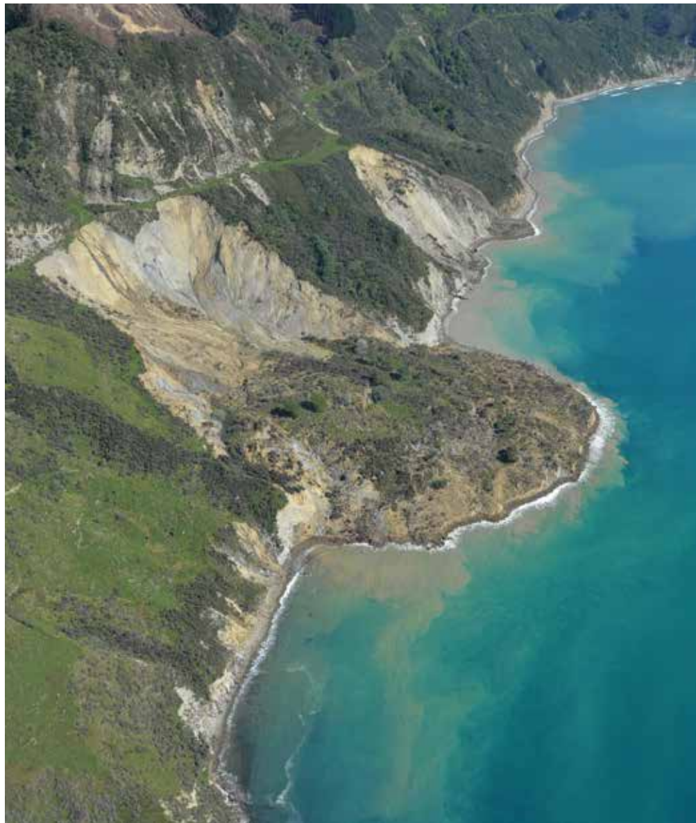
Whareongaonga landslide near Gisborne
