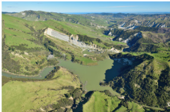
c) Landslide dam and drainage disruption, Te Tairāwhiti 2022
