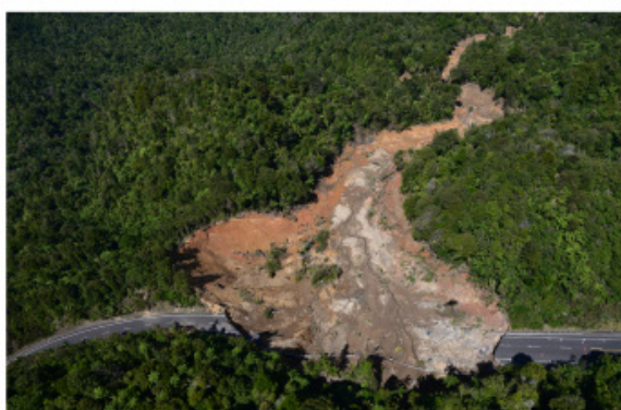
g) Undermining and disruption to SH 25, Coromandel 2023
