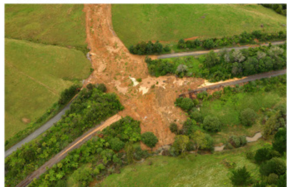
f) Inundation and disruption to railway and road, Auckland 2023
